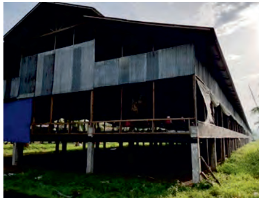
Figure 9.6. High Rised Poultry House.
