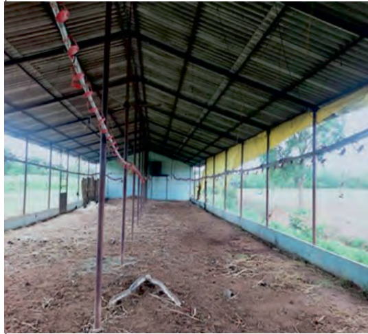
Figure 9.4. Poultry house with two open sides.
