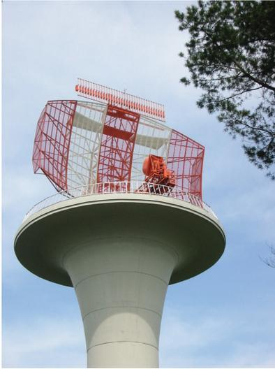
(a) Radar antenna. The parabolic antenna is the PSR and the rectangular one above it is the SSR. © Magnus Manske / Wikimedia Commons / CC-BY-SA-3.0.
