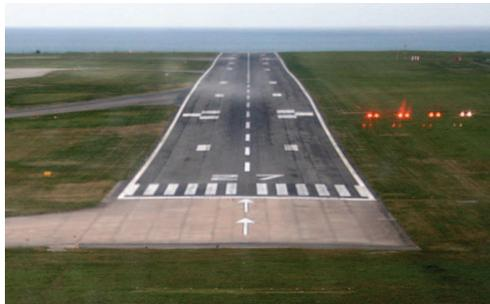
Figure 9.14: PAPI: The greater number of red lights visible compared with the number of white lights visible in the picture means that the aircraft is flying below the glide slope. [Wikimedia Commons](#) / Public domain.
