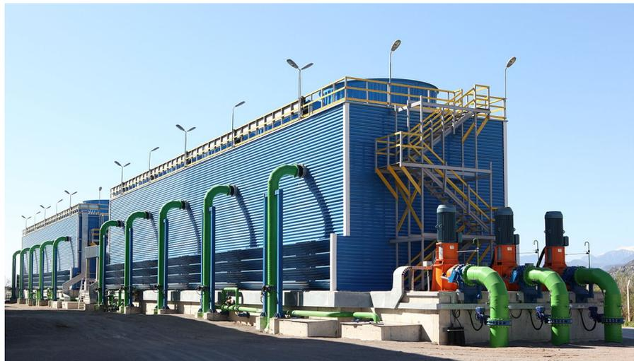
Figure 9.8: A condenser in which the heat is dissipated directly into the atmosphere, by forced convection using fans.
