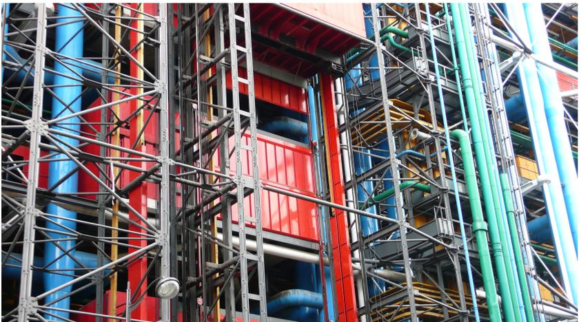
*Figure 3-9: Hinged (pinned) connections in the structure of George Pompidou Center*
