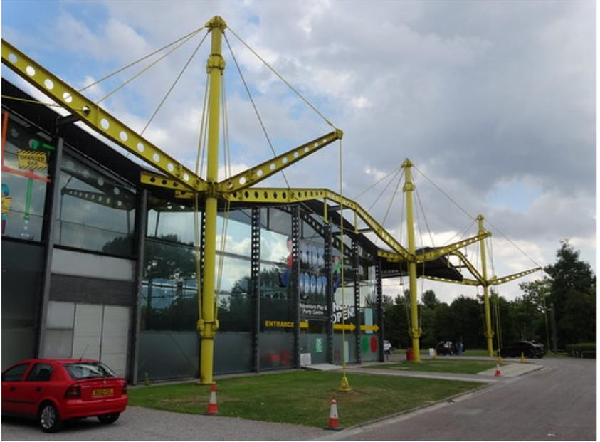
*Figure 3-8: Hinged (pinned) connections in the structure of Renault Center in Britain*
