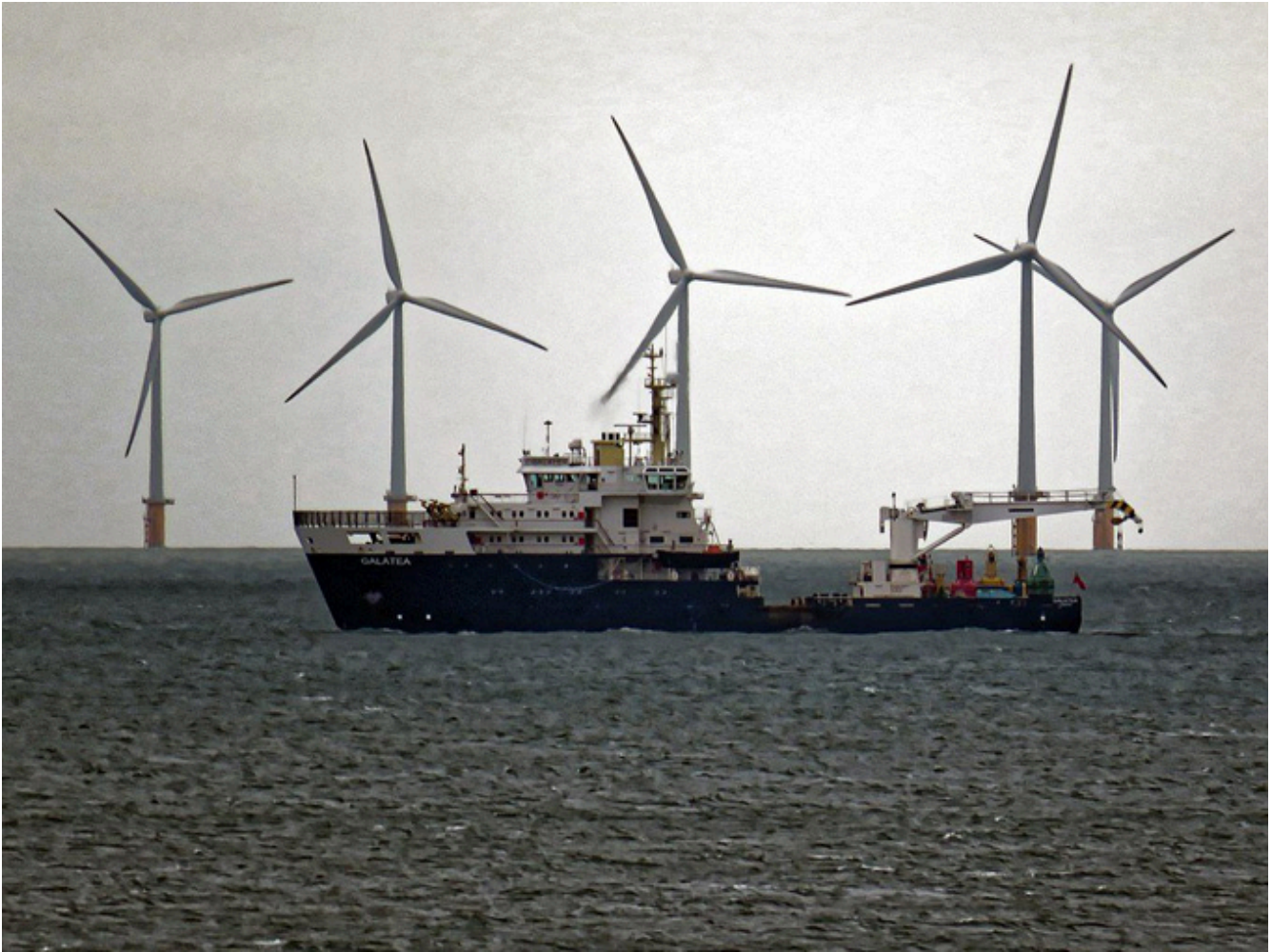
Figure 8.1 Cable ship deployed to support offshore wind energy generation and transmission to shore. CC-BY-SA by Acabashi.
