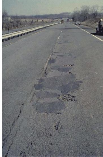
*Figure 3.14 - Patching in Asphalt Pavements*
