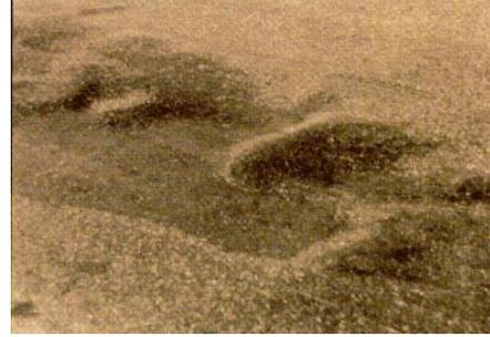
Figure 3.12 - Distortions in Asphalt Pavements
