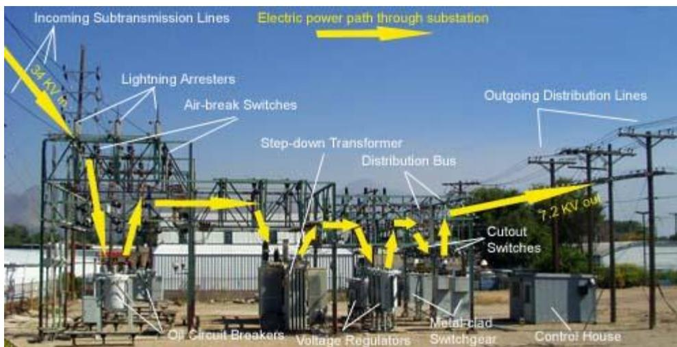
Figure 15.8 -Components of a Typical Substation
