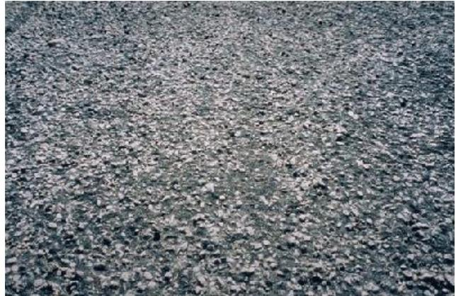
Figure 3.16 - Weathering and Raveling in Asphalt Pavements
