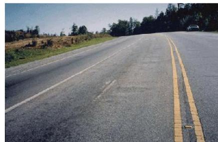
downward displacements in the pavement surface, series of closely spaced ridges and valleys, or localized longitudinal displacements of the pavement surface.
