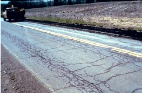
Alligator cracking is a series of interconnecting cracks caused by fatigue of the asphalt concrete surface under repeated traffic loading.
