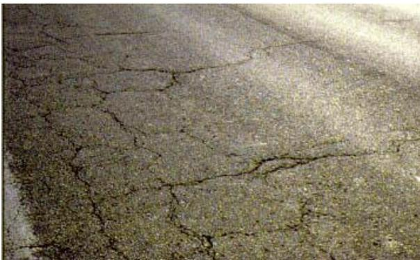
Blocks are interconnected cracks that divide the pavement into rectangular pieces. Block cracking usually indicates that the asphalt has hardened significantly.
