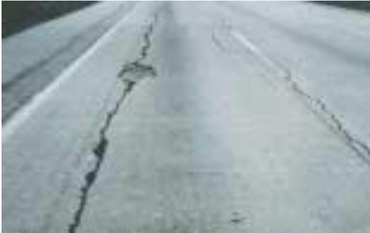
*Figure 2.3 - Example of longitudinal cracks affecting condition rating on a roadway segment*
